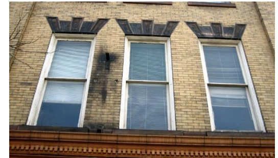
Before - Wood windows deteriorated beyond use.
