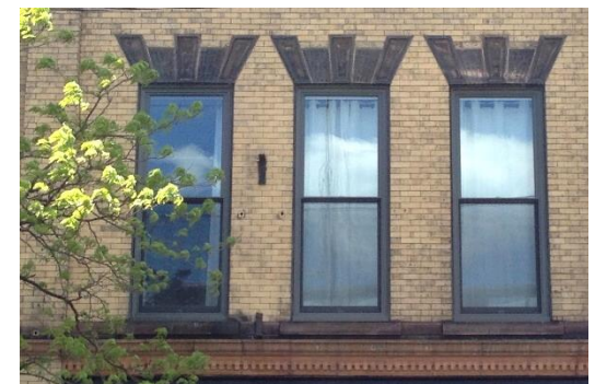
After - Windows were replaced with aluminum clad wood windows that matched the original configuration, profile, and setback.
